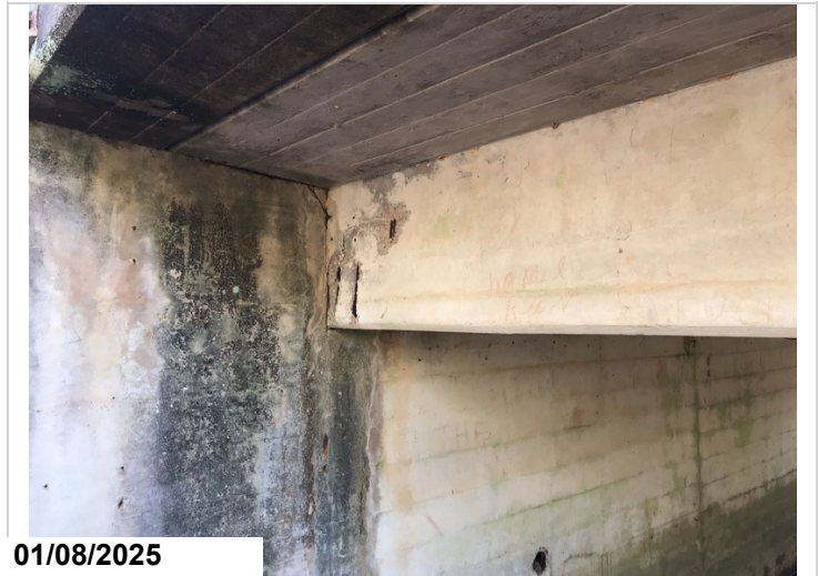
Girder 1, left side at bent 3: spall with exposed rebar. CS3-2'
