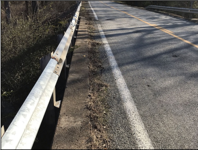
Dirt and debris accumulated in the gutter line
