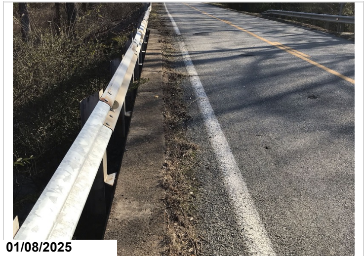
Dirt and debris accumulated in the gutter line
